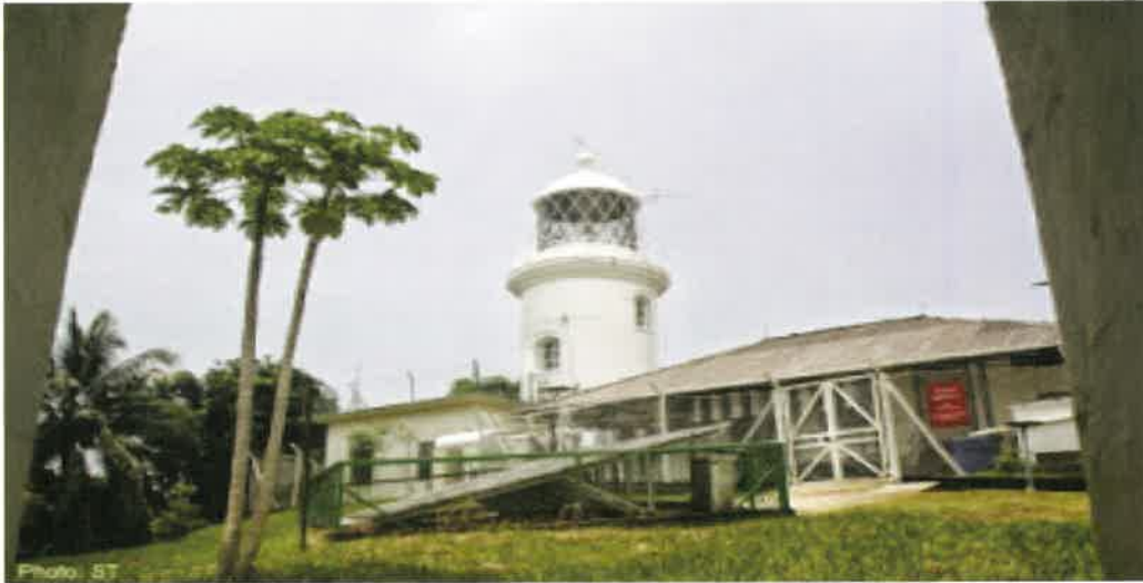
Photo 2: Photo of Pulau Pisang Lighthouse
